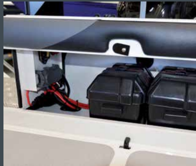
Dual batteries with isolation switch. Don't go offshore without two batteries
